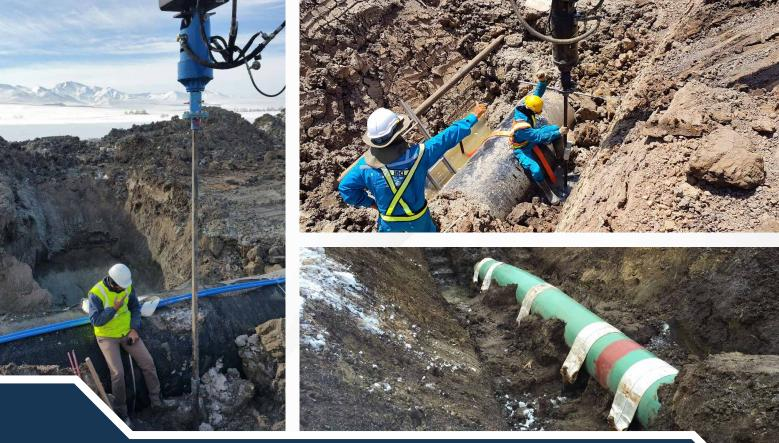
Cyntech's Pipeline Anchor System provides more than 50% construction cost savings when compared to traditional buoyancy control methods. Cyntech has over 100,000 pipeline anchor systems in service, stabilizing over 4,000 km of large diameter pipelines worldwide.
