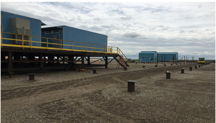
Canada - Elevated, modular buildings supported on helical piles
