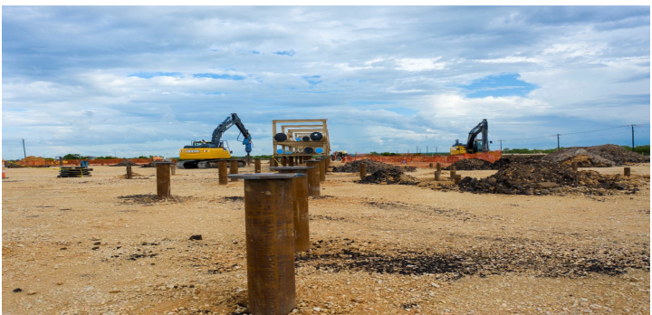
Texas - Helical piles expedited construction of this modular piperack
