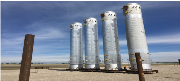
Canada - Custom steel grillage eliminated concrete
