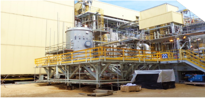
Russia - Process module supported on helical piles
