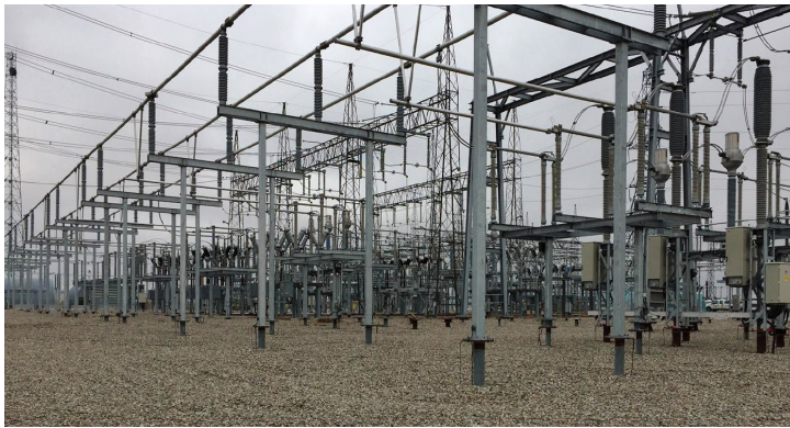
Substation supported by helical pile foundations with steel-to-steel connections.
