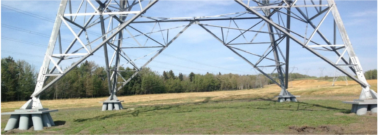
Cyntech designed and supplied helical piles for 137 lattice tower structures.
