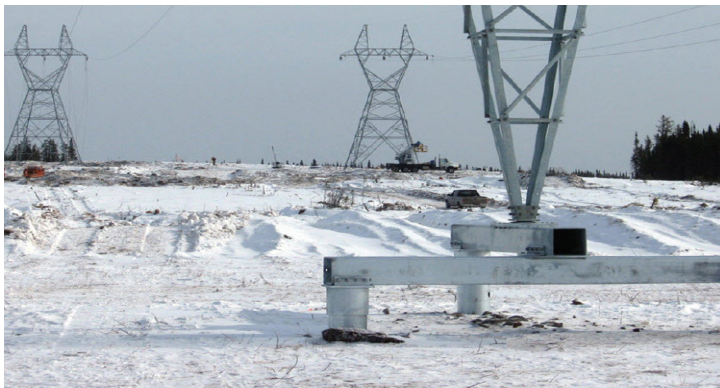
Guyed-V tower supported on helical piles with a steel-to-steel connection with no welding required.
