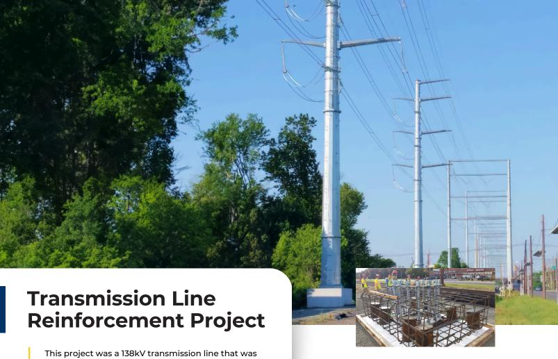
This project was a 138kV transmission line that was being upgraded to a 230kV transmission line.
